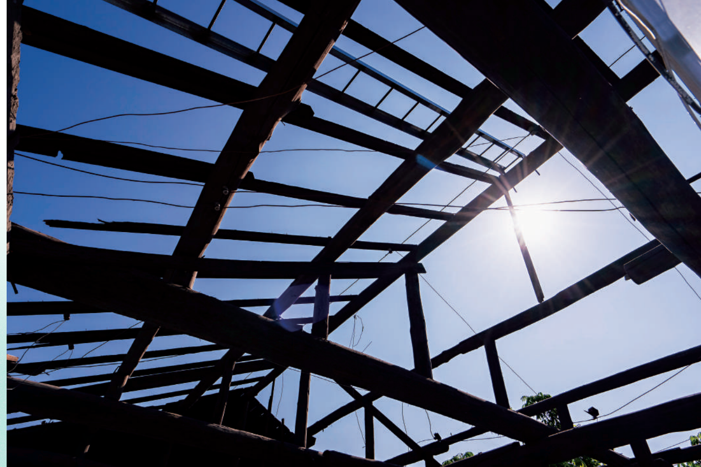
▲ 屋瓦拆除後的房子 The house after the roof tiles were removed.
