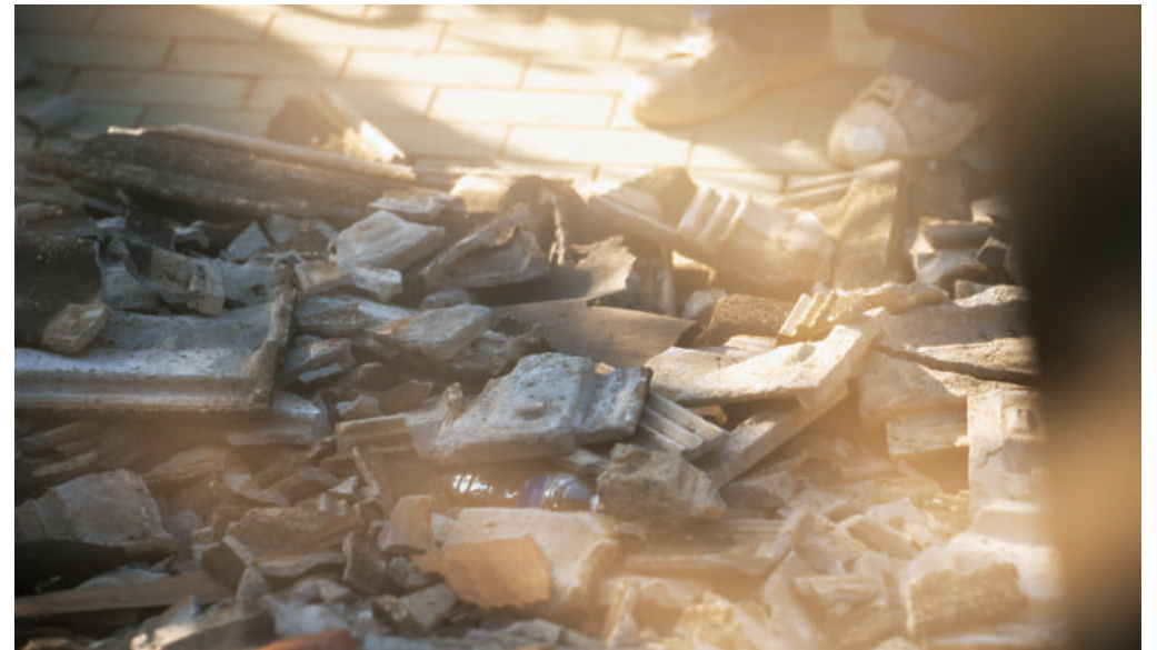
▲ 碎裂的屋瓦 Broken roof tiles.
